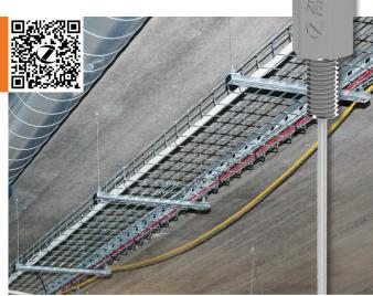
DESIGNED FOR STATIC LOADS THAT ARE SUPPORTED VERTICALLY
